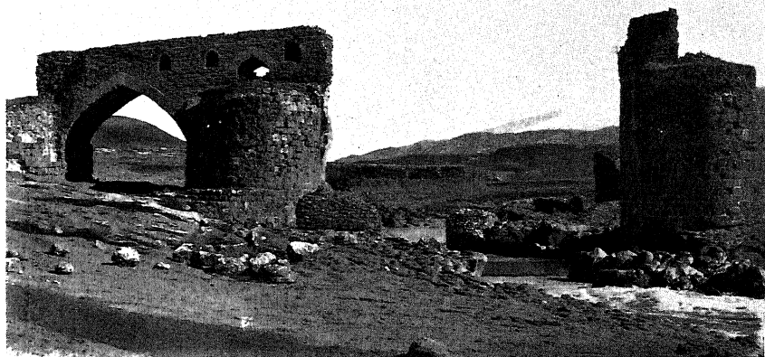
62. PIERS AND ARCH OF RUINED BRIDGE ACROSS KĀSHGĀN RIVER, AT GAUMĒSHĪ
